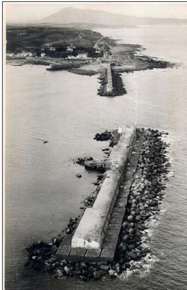
**Figure 2. Aerial view of the Artha (North, on the foreground) and Socoa (South, on the background) breakwaters, showing 50t concrete units displaced onto the parapet of the Artha breakwater after a storm in 1951 (source: Conseil Général 64).**
